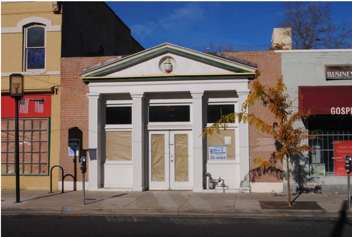
Douglass Undertaking Company, c. 2013
