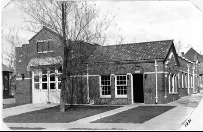
Fire Station #3, c. 1931. Courtesy of Denver Public Library, Western History Department, C Photo Album 111. Denver Fire Department
