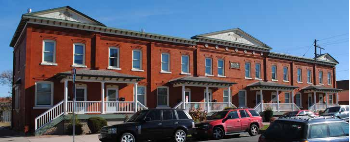
Return a Contributing Building to its appearance during the Period of Significance or its most significant period of history.
