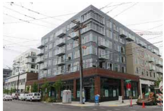
EFIS and vinyl windows are not similar quality, scale, and texture to the original facade, and are not appropriate in the cultural district.
