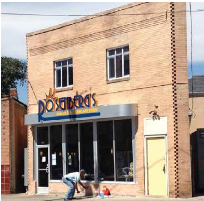
A new storefront reinforces the character-defining features
