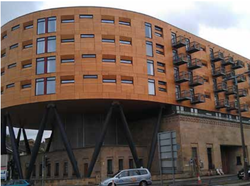
The original facade lacks prominence and is overwhelmed by the addition, and is not appropriate in the cultural district.
