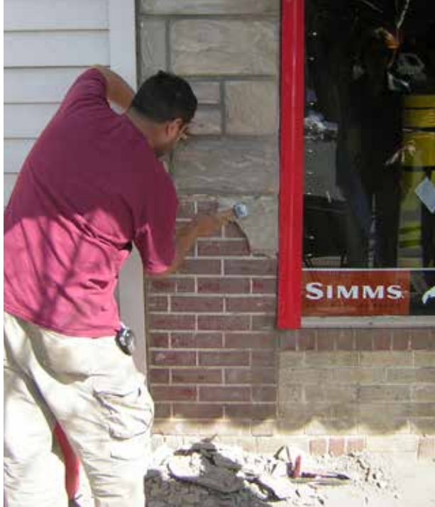
Remove stucco, or other alternative material, from brick only when testing demonstrates that this can be done without damaging the historic brick.
