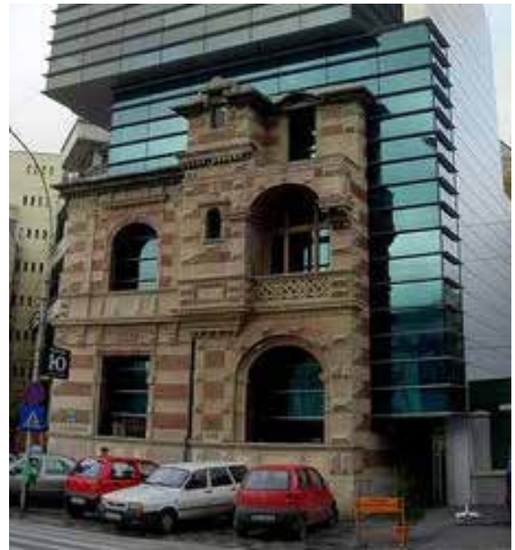
The addition lacks an articulation and scaling relationship to the original facade, and is not appropriate in the cultural district.
