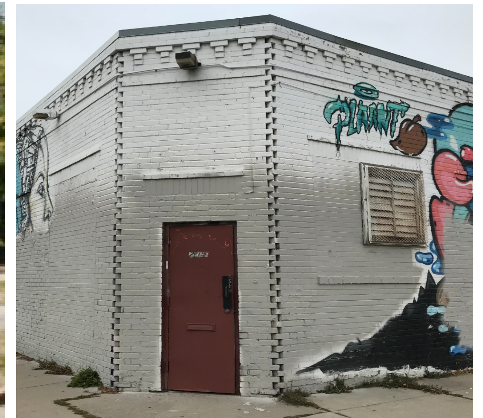
EXISTING CORNER ENTRY
